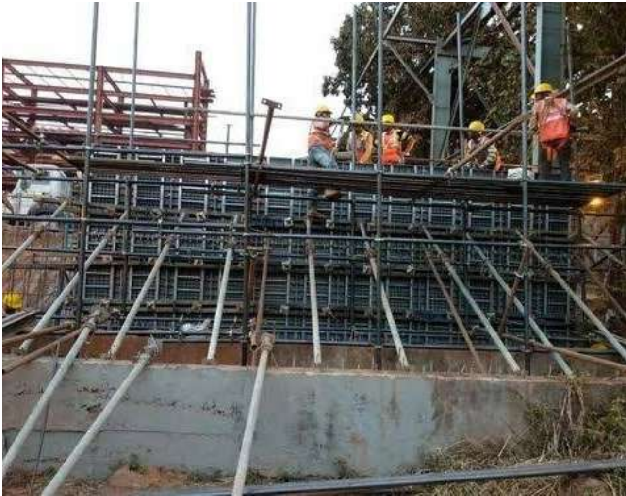
Construction of the retaining wall at in Sirsa Hisar Hariyana.
